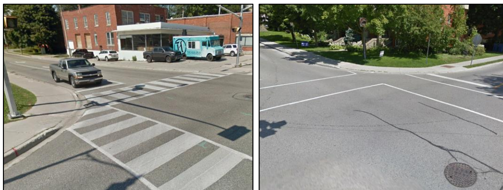
Figure 8: Typical Ladder and Standard Crosswalk Treatments
