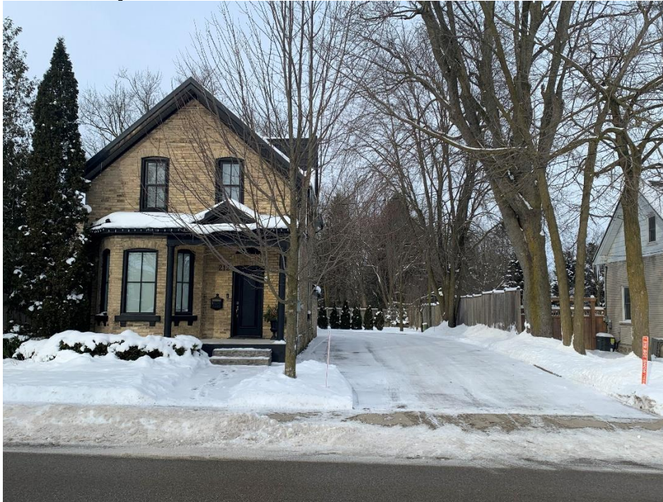
Figure 2 – Site Photo – 212 Railway Avenue (January 10, 2025) File # B09-24 John Carey-Woodman – 16 Chestnut Street
