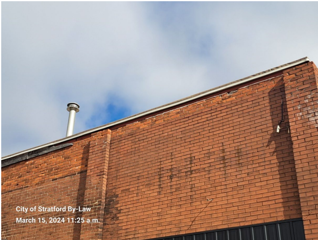
- Deteriorated/missing fascia.
