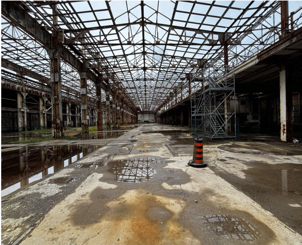
INTERIOR VIEW LOOKING WEST
