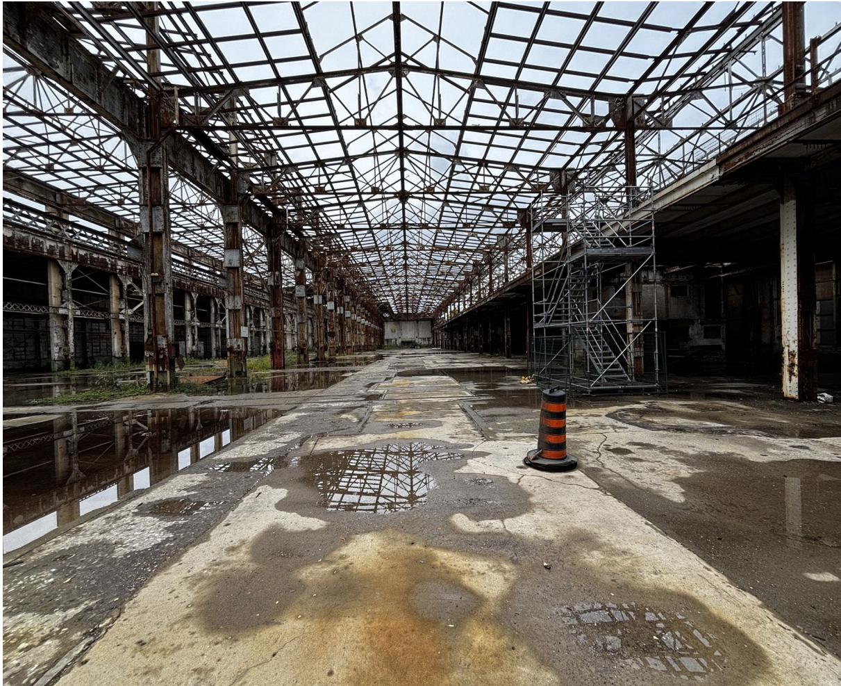
INTERIOR VIEW LOOKING WEST
