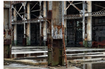
EXISTING STRUCTURE TYPICAL COLUMN BASE
