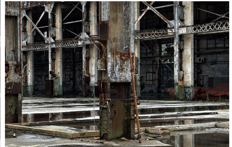
EXISTING STRUCTURE TYPICAL COLUMN BASE
