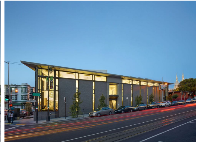
North Beach Branch Library | Leddy Maytum Stacy Architects 8,500 ft 2
