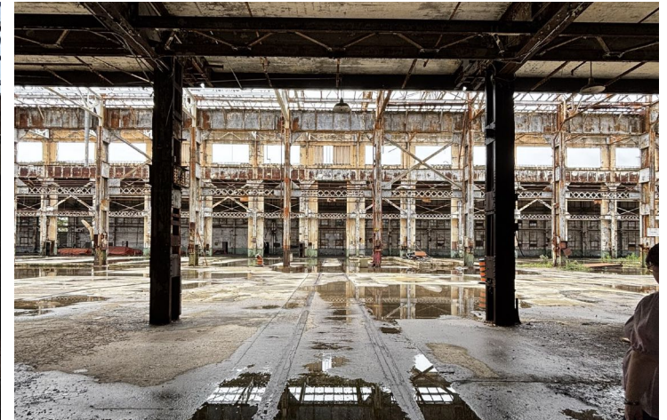
INTERIOR VIEW OF MEZZANINE FROM UNDERNEATH
