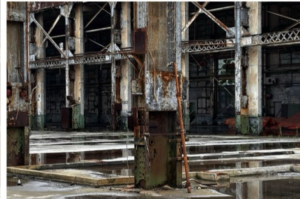
EXISTING STRUCTURE TYPICAL COLUMN BASE
