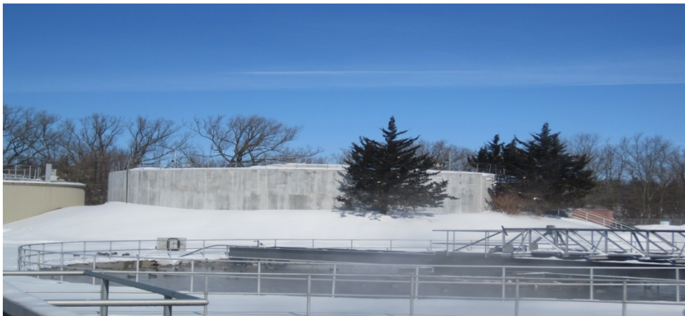
Sludge storage tank
