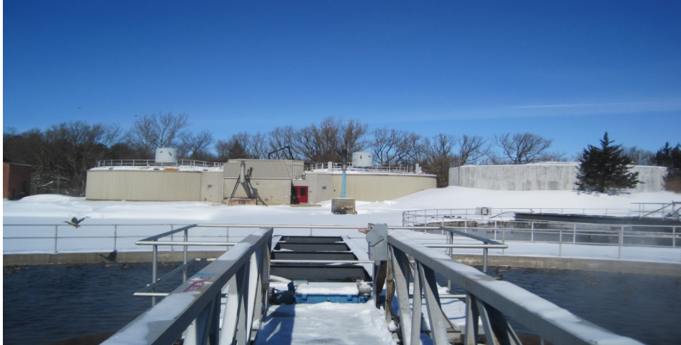
2 Stage Anaerobic Digestion (Primary on the left and Secondary on the right, boiler room in the middle)
