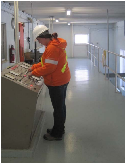
Filter control room
