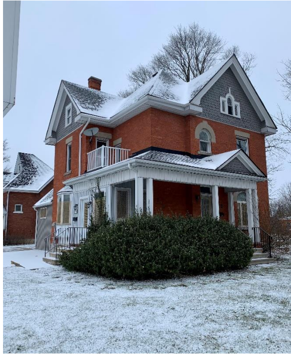
2. The commanding presence of 370 Ontario Street at the corner of Ontario and Trow streets, Hayden Bulbrook, December 2020.
