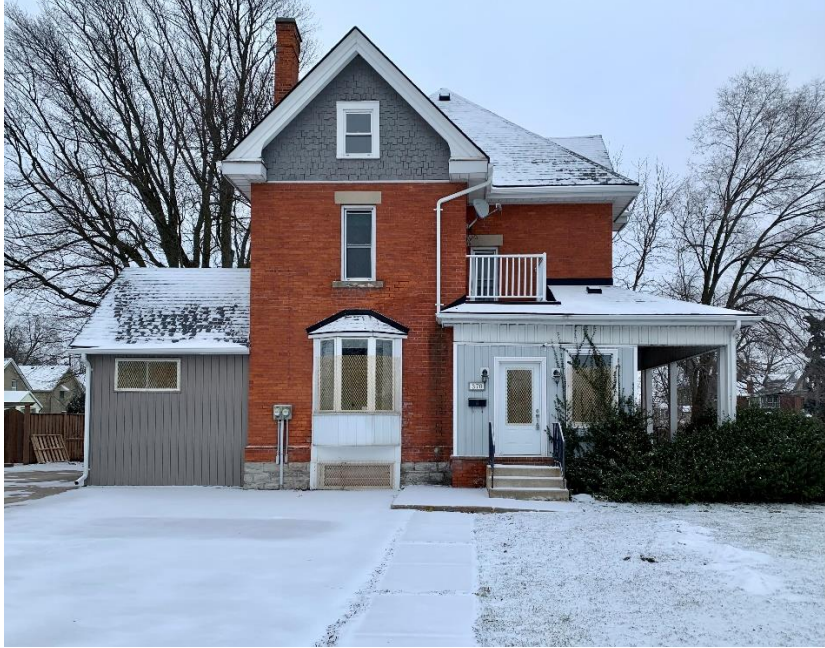
1. West view of 370 Ontario Street. Note the stone lintels, brick chimney, staggered shingle patterned gable, rich red brick and sympathetic bay window, Hayden Bulbrook, December 2020.
