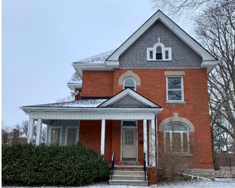
3. 370 Ontario Street from Ontario Street. Note the stone arches and lintel, staggered shingle patterned gable, Hayden Bulbrook, December 2020.
