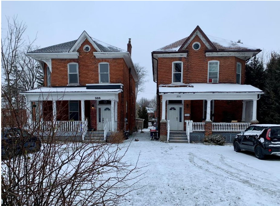
4. 388 and 390 Ontario from Ontario Street. Note the symmetrical building plans and similar features, Hayden Bulbrook, December 2020
