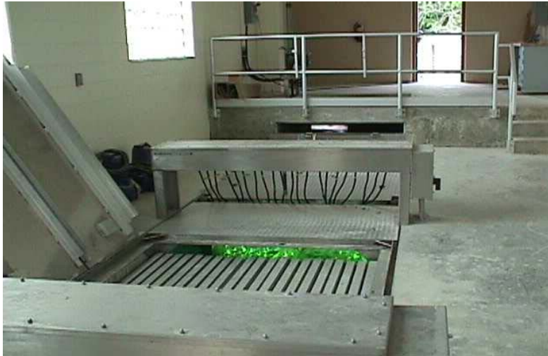
Figure 12: Ultraviolet Disinfection
