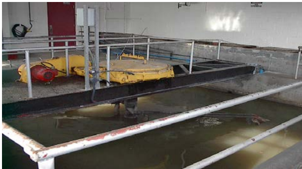
Figure 4: Grit Removal System
