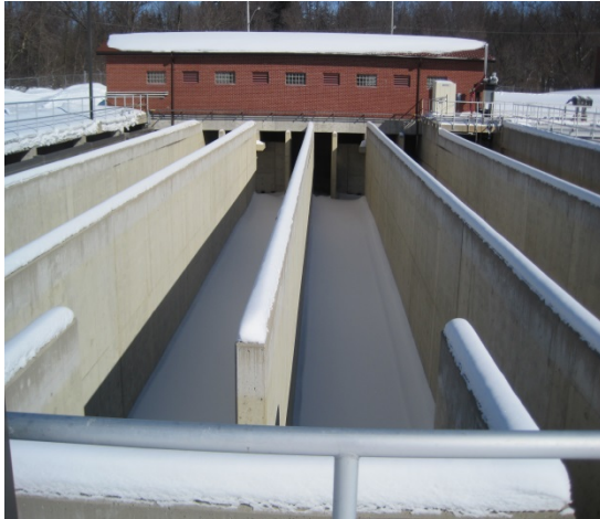
Figure 1: Chlorine Contact Chamber
