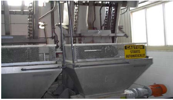
Figure 3: Automatic Bar Screens
