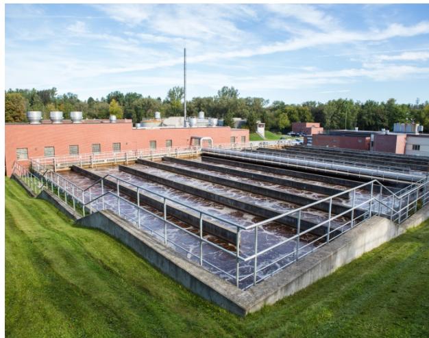
Figure 6: Aeration System
