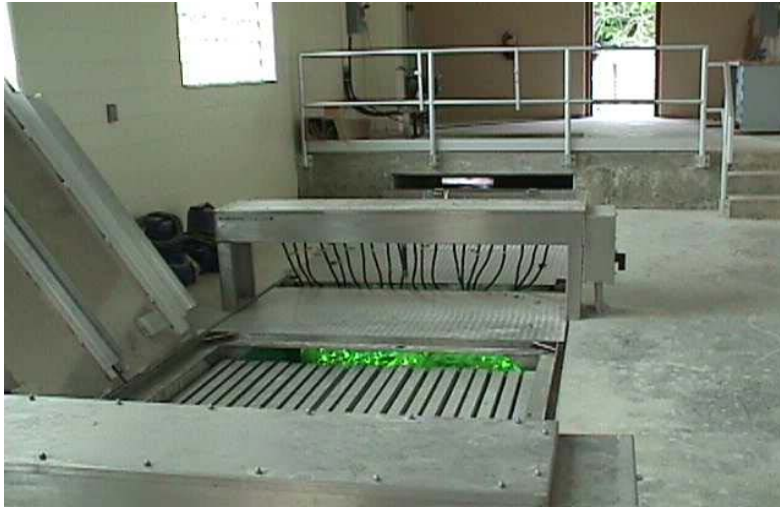
Figure 12: Ultraviolet Disinfection
