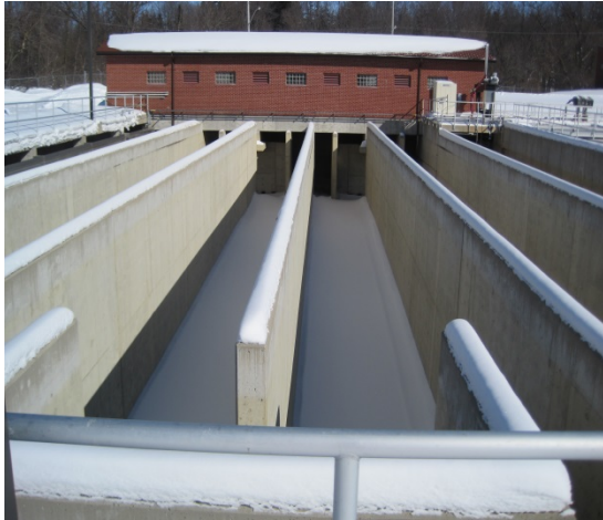
Figure 1: Chlorine Contact Chamber
