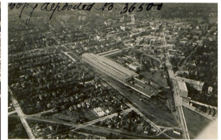
HISTORICAL AERIAL OF GRAND TRUNK SHOP
