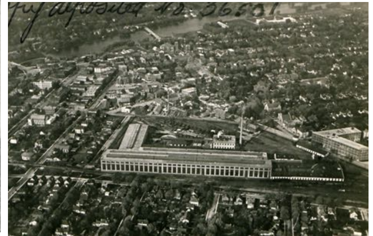
HISTORICAL AERIAL OF GRAND TRUNK SHOP
