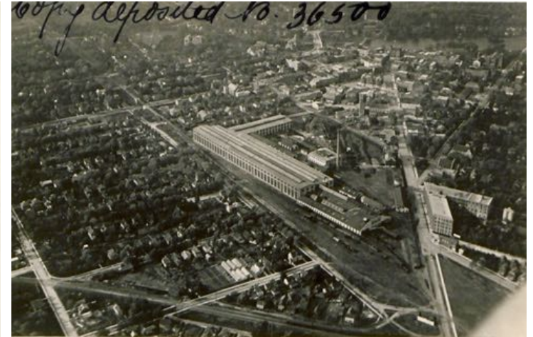
HISTORICAL AERIAL OF GRAND TRUNK SHOP
