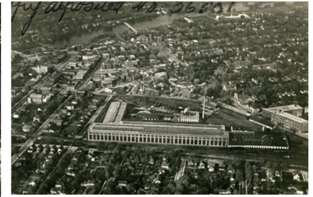
HISTORICAL AERIAL OF GRAND TRUNK SHOP
