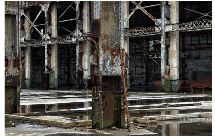
EXISTING STRUCTURE TYPICAL COLUMN BASE
