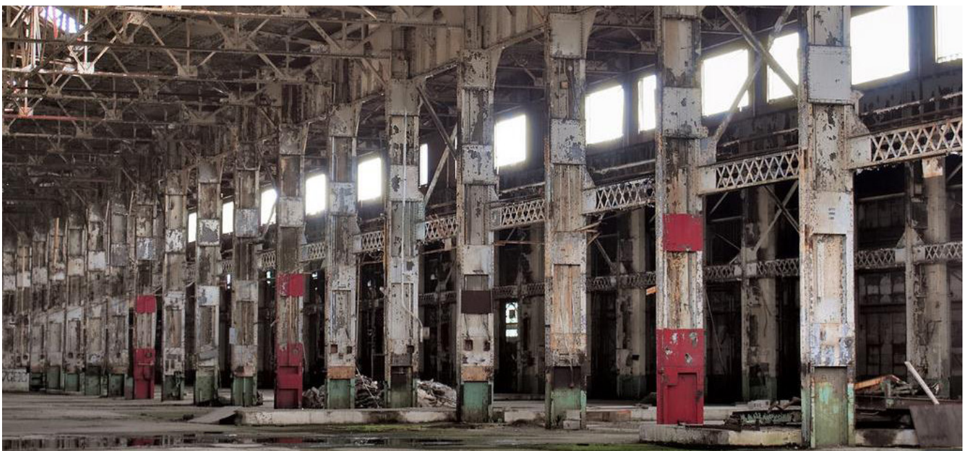
Figure 19 ► Grand Trunk Building interior
